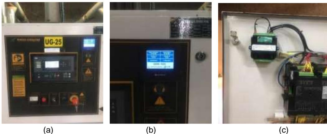
**Figure 9.** PLC operating in the panel of the generating unit #25: (a) general panel of unit #25, (b) new display included in this development, and (c) connections of the slave CLP.
