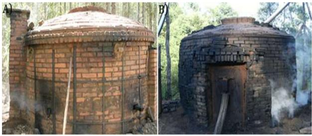
**Figure 2** – A) Hot-tail oven with chimney. B) Brochier oven *Figura 2* – A) Forno rabo-quente com chaminé. B) Forno Brochier
