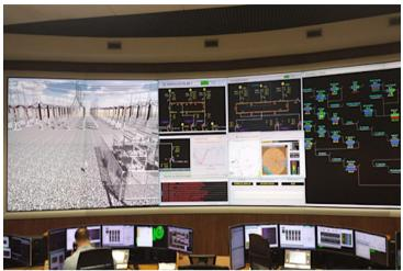
**Figure 3.** Virtual Reality System for substation operation shown on the left side of the display.
