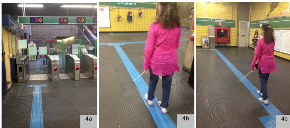
Figure 4 - (a) Access to the subway station; and (b) and (c) tactile track directions
