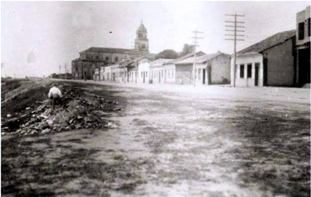
Figure 2 –São José Street following the expropriation, 1939-1940.
