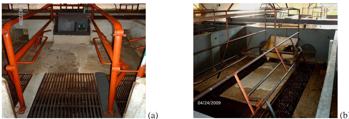
FIGURA 2. Celas maternidade confeccionadas em alvenaria (a) e placas de ardósia (b). Farrowing stalls built with masonry (a) and masonry slate boards (b).
