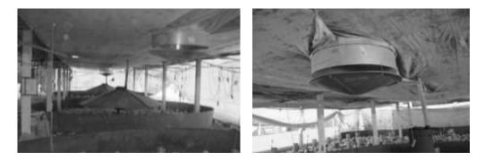
FIGURE 1. Minimum ventilation system by positive pressure (ventilator). Ventilator positioned inside the installation on the lining height, with coupled deflector in order to avoid the incidence of air jet directly on the birds.
