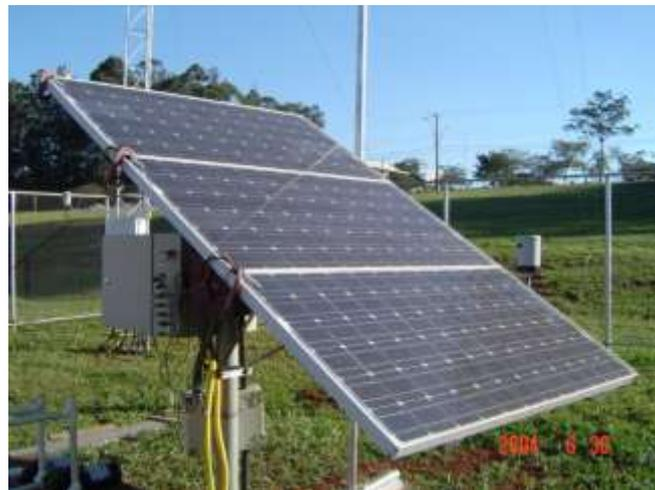
FIGURE 3. PV modules of 100 Wp each, installed in parallel and constituting the photovoltaic panel system installed at the Laboratory of Rural Energization of FCA/UNESP.
