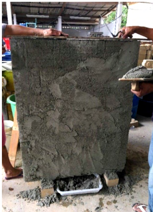
Figure 5: Masonry of ceramic blocks coated with mortar with scheelite residue.
