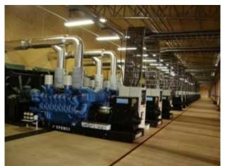
Figure 8. Part of the 99 generating units of the Palmeiras de Goias Thermal Power Plant.
