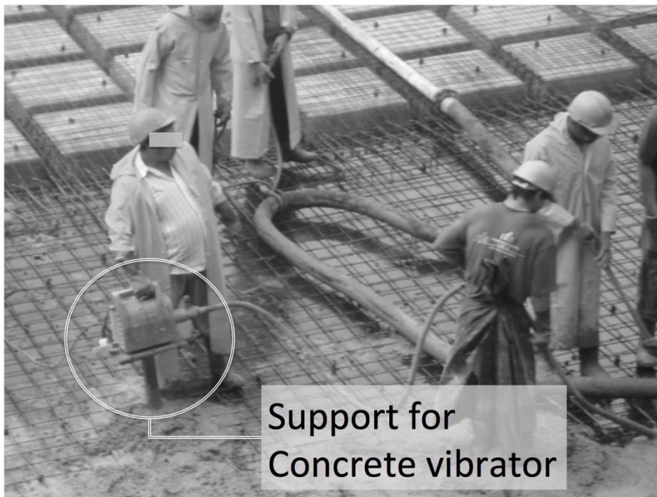
Figure 3 - Improvisation for improving ergonomic conditions of concrete pouring
