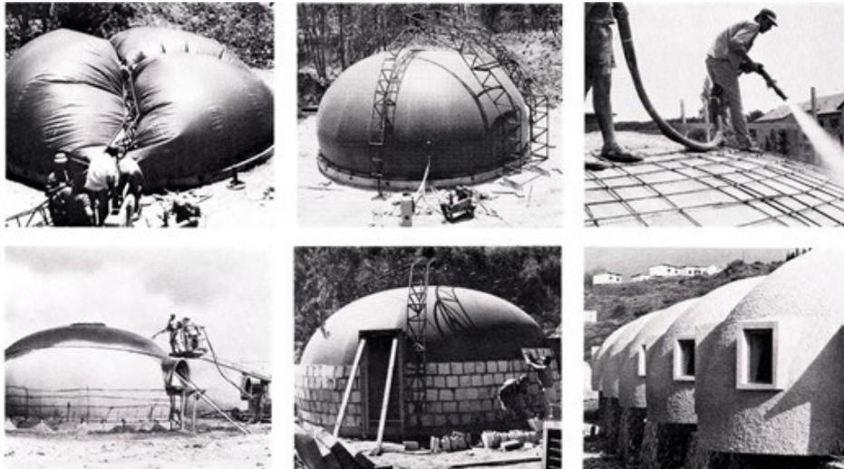
**Figure 13.** Stages of construction of the Domecrete Building System. Adapted from [31].
