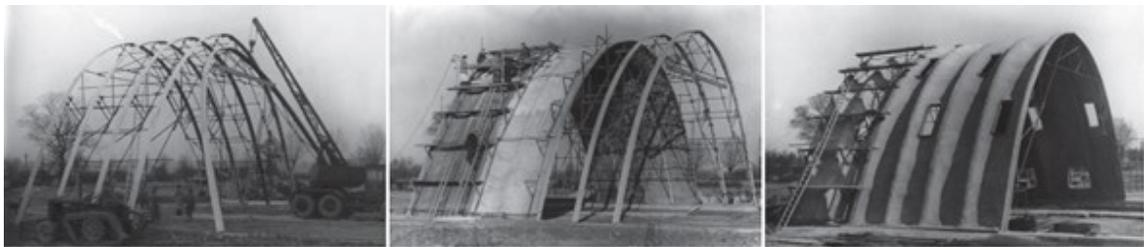
Figure 6. Construction process of the “Ctesiphon” system. Adapted from [6].
