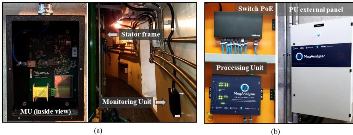
Fig. 15. Equipment installation: (a) monitoring unit, (b) processing unit and PoE switch on the external panel.
