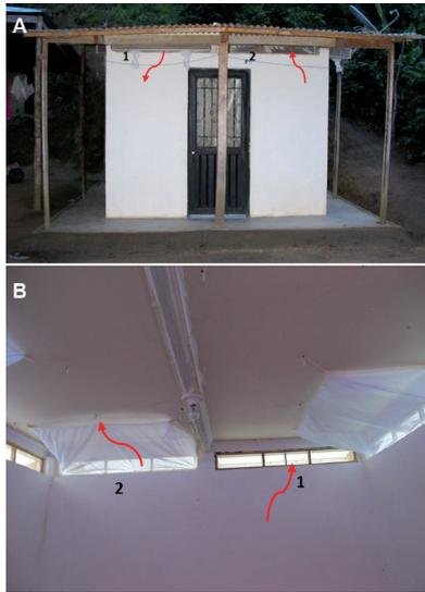
Fig. 3: image of the experimental hut. (A) external view showing the front of the horizontal-slit eave exit trap (1) and entering baffle (2), and (B) traps viewed from the inside (arrows show entry and exit movements of sand flies).
