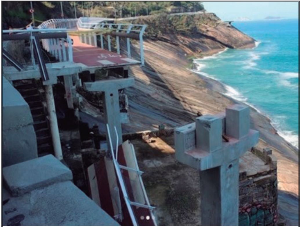
Figure 1 – Collapsed portion of the Ciclovía Tim Maia
