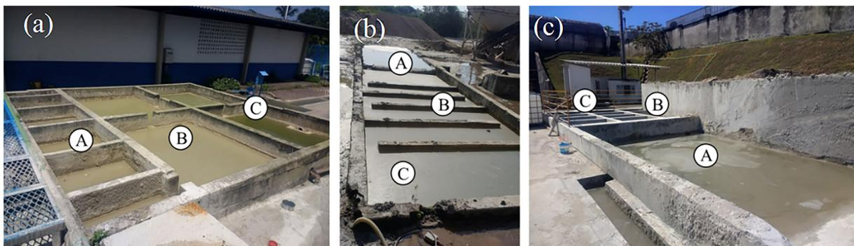
**Figure 1.** Sedimentation tanks, (a) CBP K; (b) CBP P and (c) CBP S. Collection points: (A) tank inlet, (B) tank middle and (C) tank outlet.
