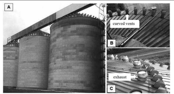
Figure 1 - Vertical metallic warehouses (A) 30m high and 26m diameter, full of bulk soybean, with curved vents on the roof (B) and with vent + exhaust system (C), Ponta Grossa – PR.
