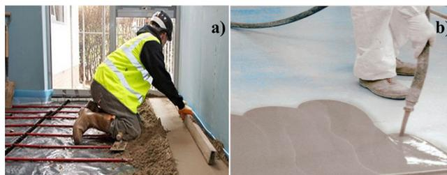
Figure 1: Images of traditional semi-dry cementitious screed (a) and self-leveling mortar (b) [5].
