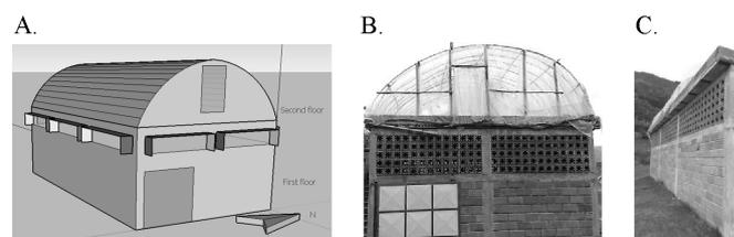
Figure 1. 3D geometry of the building: postharvest plant (first floor) and solar dryer of coffee (second floor) (A), front facade (B), side facade (with windows in perforated brick) (C)
