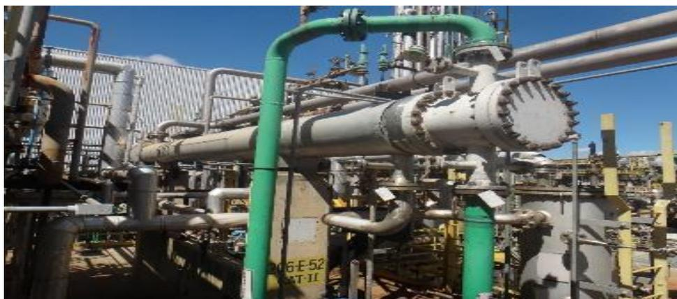
**Figure 2:** Heat exchanger of the top system of the DEA regenerating tower.
