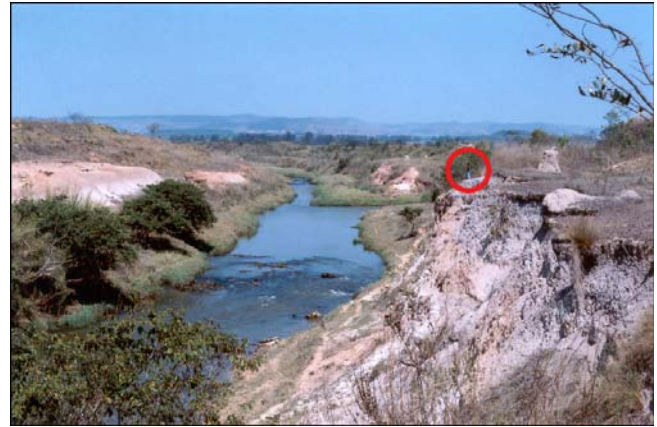
Fig. 4. Transposition canal (foreground) connecting rio Piumhi (formerly part of Paraná system) and Ribeirão da Água Limpa (São Francisco System), downstream from junction of artificial canals draining upper course (right) and reversed lower course (background) of rio Piumhi. Relative height of excavation may be estimated from size of adult person standing on top of left bank (indicated by red circle).
