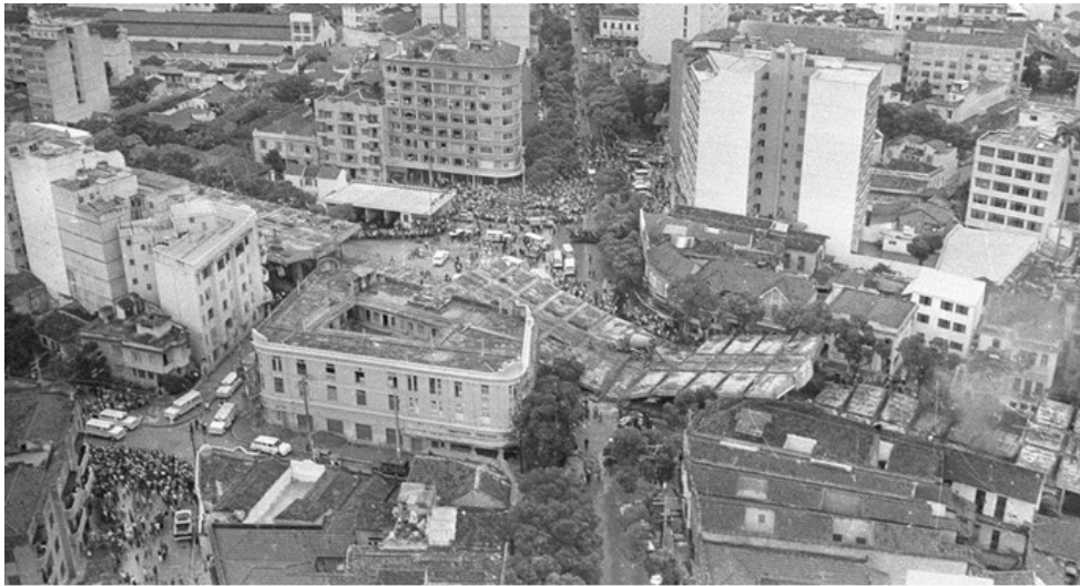
Figure 1. Collapse of Paulo de Frontin bridge.
