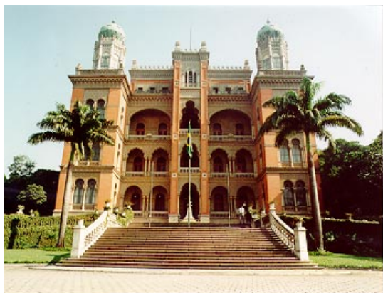
Fig. 1: main building of the Oswaldo Cruz Institute
