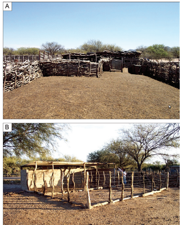
Fig. 2A: typical structure of traditional goat corral, with walls of stacked branches; B: structure of the yard with new design, concrete wall, wire and tin roof.
