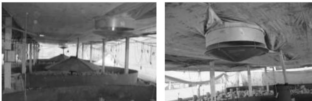
FIGURE 1. Minimum ventilation system by positive pressure (ventilator). Ventilator positioned inside the installation on the lining height, with coupled deflector in order to avoid the incidence of air jet directly on the birds.
