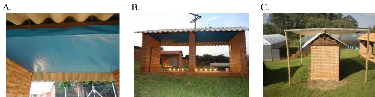
FIGURE 2. Internal view of the model with lining (A), side view of the model with lining under the fiber-cement roof (B), and frontal view of the model with lining above the fiber-cement roof (C).
