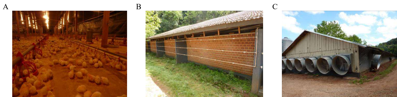
FIGURE 3. (A) Internal view, (B) external view, and (C) detail of exhaust fans in the dark house system aviary.
