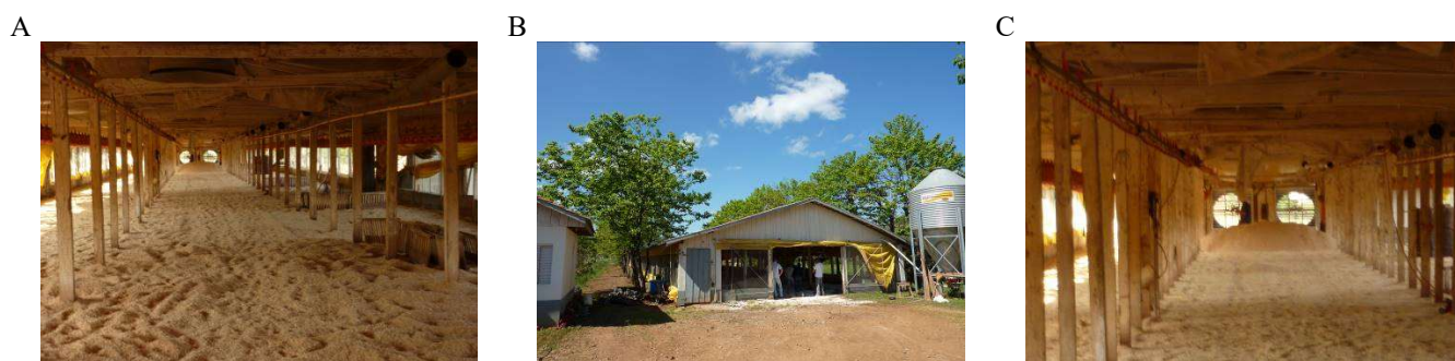
FIGURE 2. (A) Internal view, (B) external view, and (C) detail of exhaust fans in the negative Pressure system aviary.
