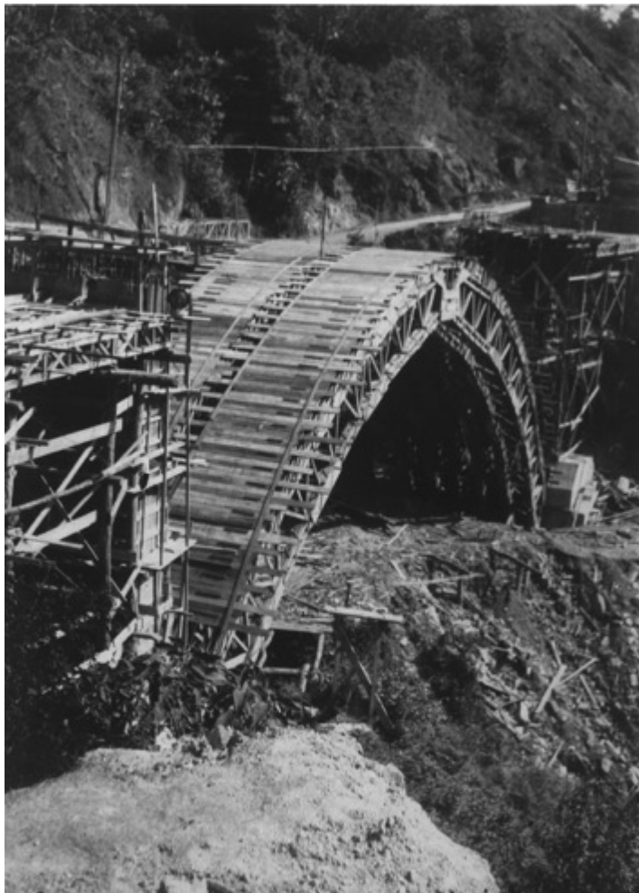
Figure 4: Bridge over Rio Tietê. Iron structure assembly (1902-1903). Unknown author. Source: Museu da Companhia Paulista (Jundiaí, SP, Brasil).
