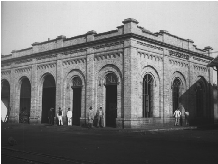
Figure 12: Power plant in Ribeirão Preto. Mogiana Company. Unknown author.
