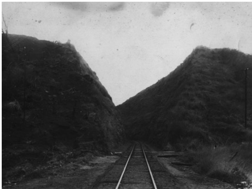
Figure 8: End of the Jaú branch rectification, Serra de Brotas segment (c.1930). São Paulo Company. Unknown author.
