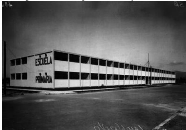
Image 4. Emiliano Zapata Elementary School, 1933.
