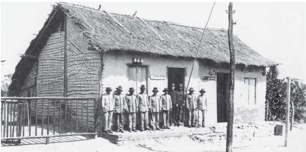
Figure 6: Juruena Station. Photograph, José Louro (Lasmar, 2008, p.80, fotografia 51)
