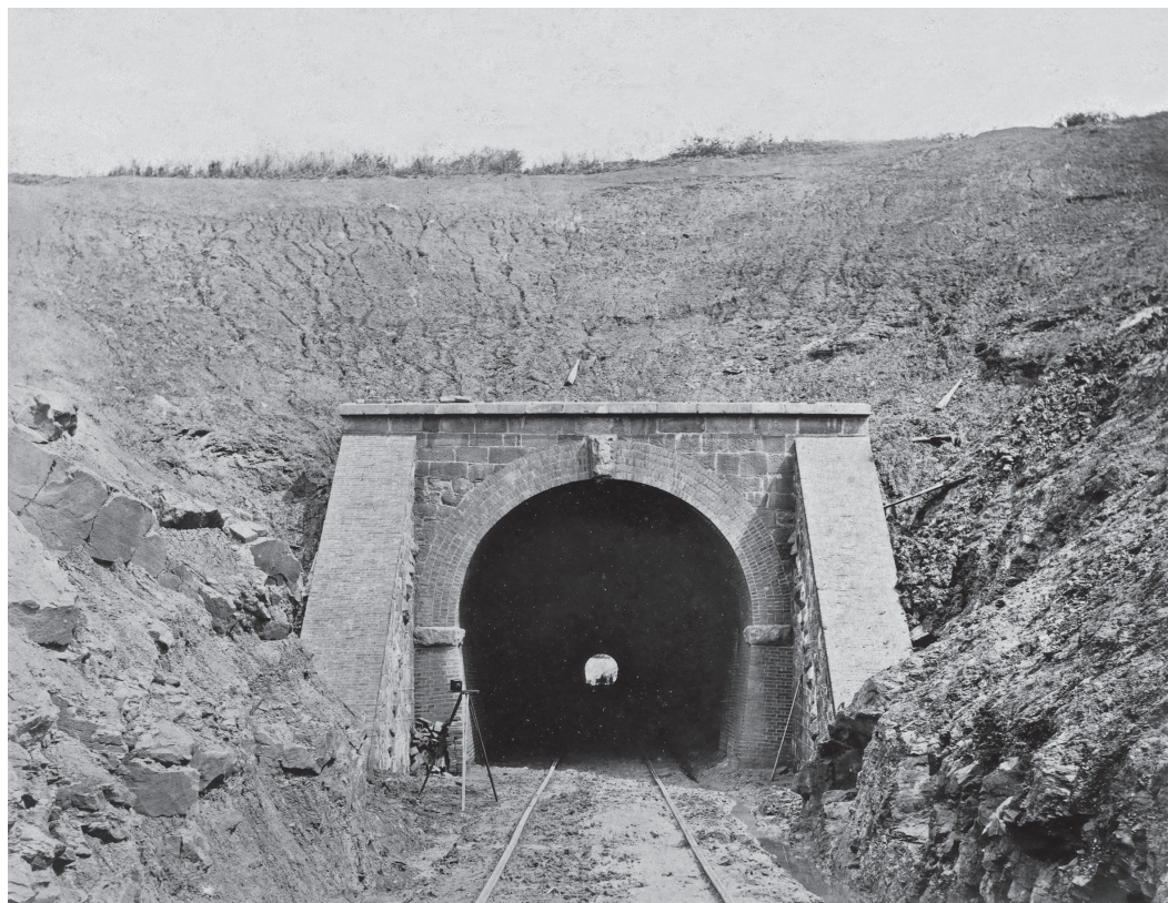
Figure 3: Benjamin R. Mullock, Entrance to Mappelle Tunnel: Bahia and San Francisco Railway (1859-1861); albumen print on paper, black and white (Coleção Thereza Christina Maria, Biblioteca Nacional)
