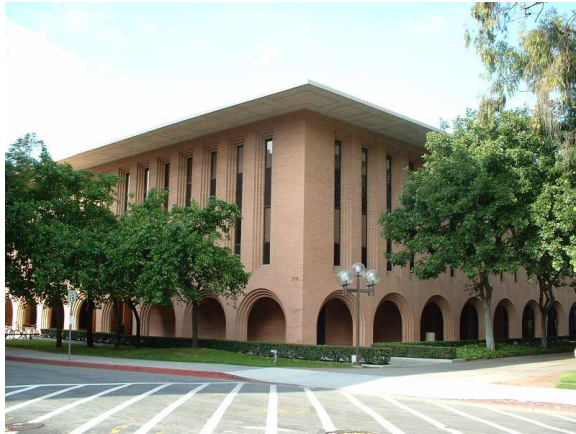
(a) USC Gerontology building
