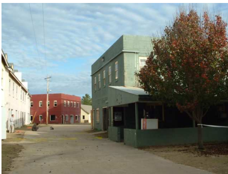
(c) Actual balcony building
