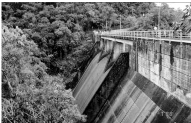
Figure 1: Downstream face of the Guaricana hydroelectric power plant dam.
