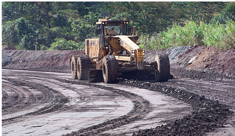
Figure 8 Scraping or grading operation on a main road.
