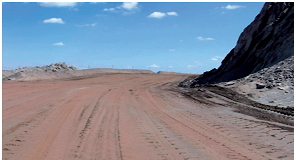
Figure 2 Irregular grade in a main road.
