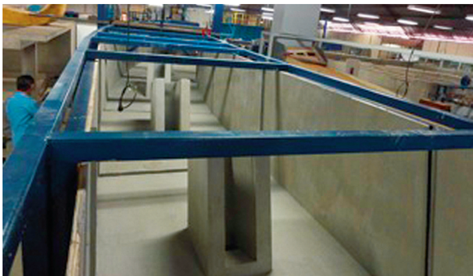
Figure 5 Water reservoir and towers already waterproofed with SikaTop.
