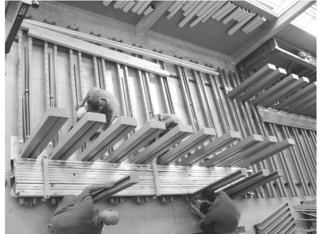
Pressing of the beam.
