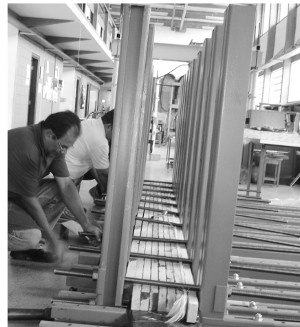
Pressing of beam with reinforcement.
