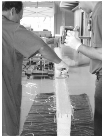
Application of fiberglass fabric.
