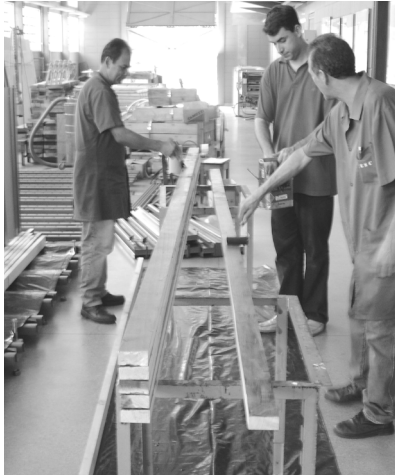
Application of glue on sheets.
