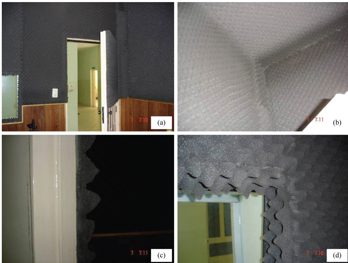
Figure 2. Location of the assembly of the experiment; (a) Rehearsal studio; (b) Coating on superior part of the room; (c) Detail of the thickness of the door; (d) Detail of the window double glazing.
