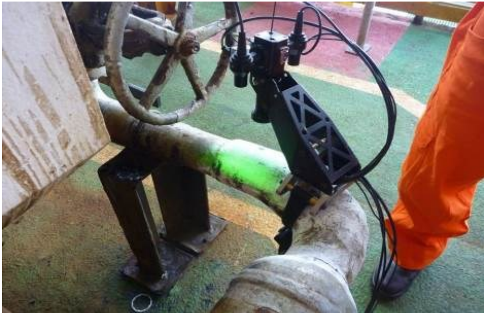
Figure 6: Shearography inspection of a composite repair in an offshore platform. The collar system was used to clamp the shearography device to the repair.
