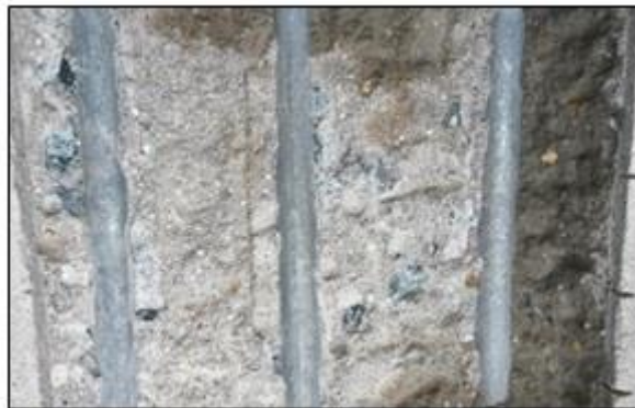
Figure 17: Galvanized tubes in the dry environment experiment (without water spray).
