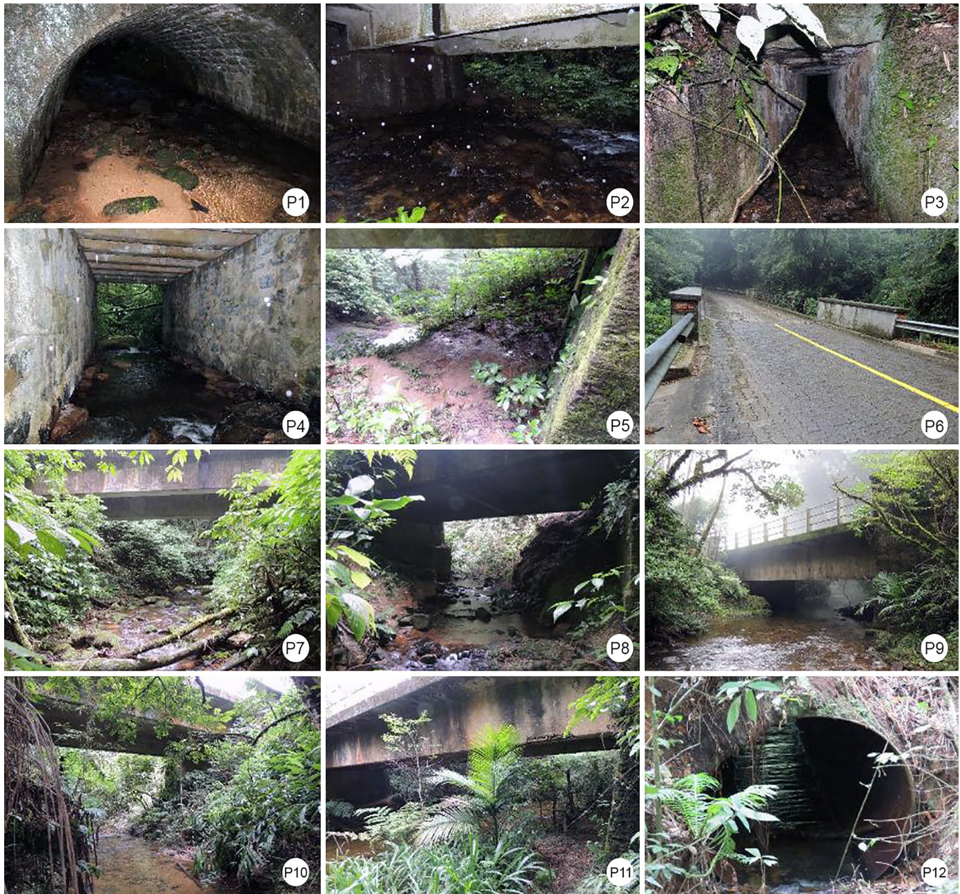
Figure 2. Existing wildlife underpasses along Serra da Macaca Park Road (SP-139). P1 – Circular culvert (Km 46+800), P2 – bridge (Km 56+200), P3 – rectangular culvert (Km 56+620), P4 – rectangular culvert (Km 58+714), P5 – bridge (Km 60+300), P6 – bridge (Km 61+300), P7 – bridge (Km 64+660), P8 – bridge (Km 67+100), P9 – bridge (Km 69+710), P10 – bridge (Km 73+850), P11 – bridge (Km 76+200), and P12 – circular culvert (Km 76+860).
