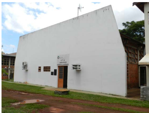
Figure 2 - East facade of the Building Materials Laboratory
