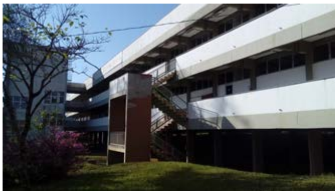
Figure 1 - North facade of the Classroom Centre
