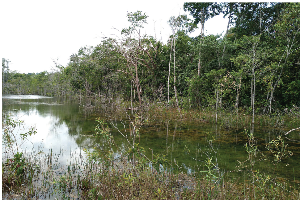
FIGURE 4 | Lagoon at the rio Mutum headwater due to the construction of a road, tributary of rio Camararé, upper rio Juruena basin, rio Tapajós basin, Comodoro, Mato Grosso, Brazil.
