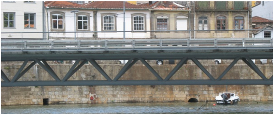
Figure 1: Example of a structure with hollow sections.
