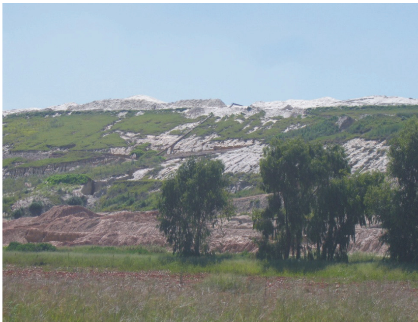
Figure 2: 'Mega-dump' of reprocessed gold tailings, south-east of Springs, Gauteng Province. Heavy rains in February 2008 led to landslides that denuded large parts of the previously vegetated slope.
