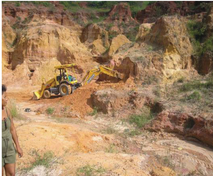
Figure 5: Initial work in areas 4-8. Source: LAGESOLOS, 2008.
