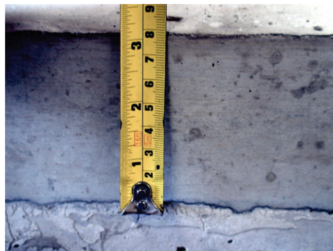
Figure 8 - Tensile layer aspect after the retrofitting and strengthening
