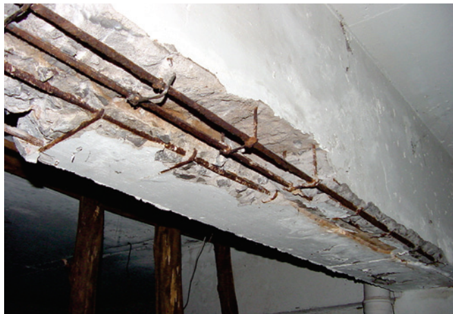
Figure 2 – RC beams with tensile zone damaged by effect of corrosion (Ferrari (5))
