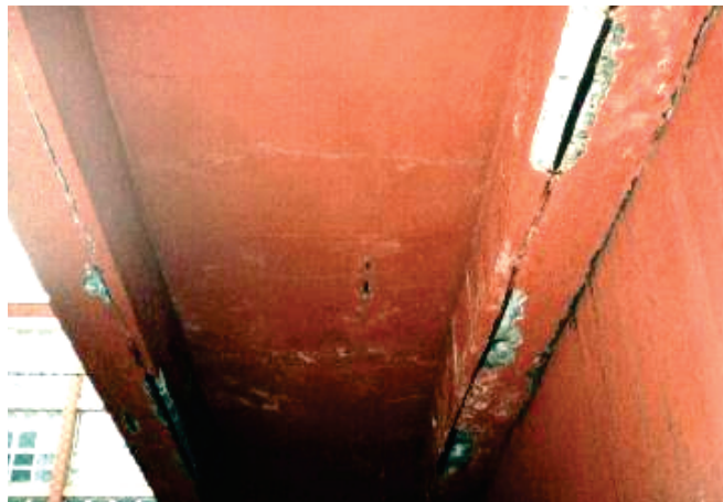
Figure 2 – RC beams with tensile zone damaged by effect of corrosion (Ferrari (5))
