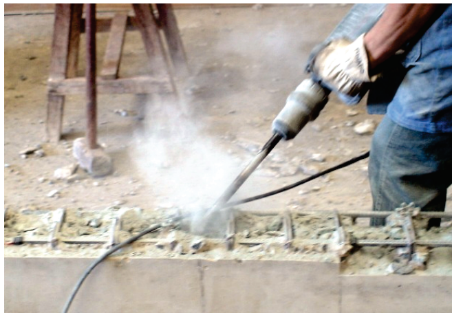
Figure 7 - Removal of concrete from the tensile zone of the beam V2C
