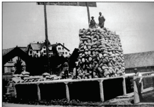
B Tests carried by Maillart (Furst e Marti (11))
