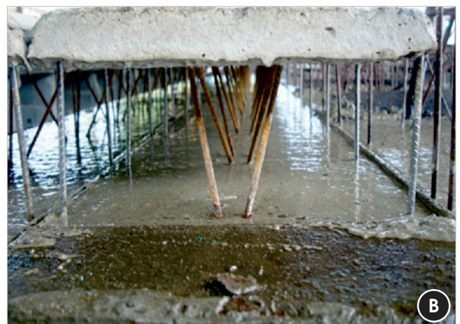
Concreting of the opposite side
