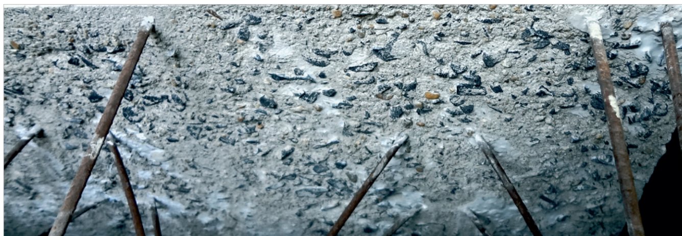
Figure 6 - Panel with exposed coarse aggregate
