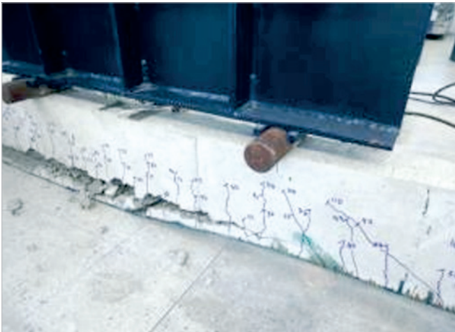
C VA-3 beam in the collapse
