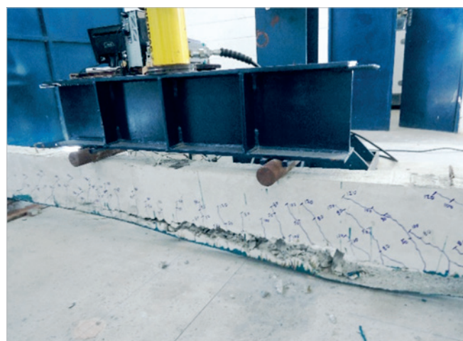
E VA-5 beam in the collapse
