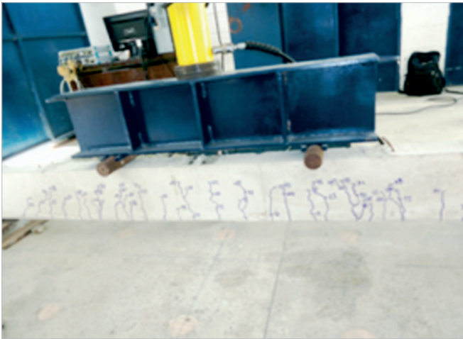
A VA-R beam in the collapse
