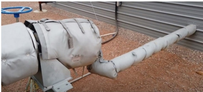
Figure 8. Pipe containing the CO 2 that will be injected into the carbonation chamber. Source: [[38]].
