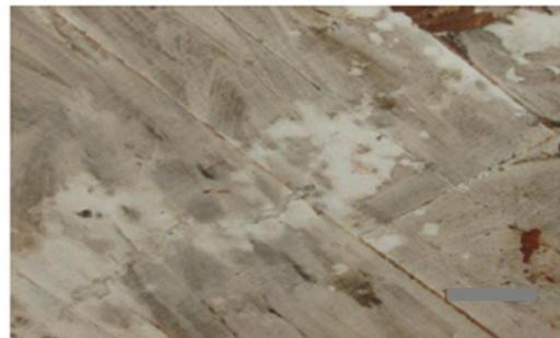
b) Deck slab with crack showing efflorescence
