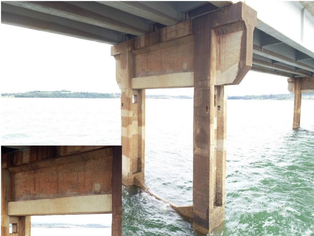
**Figure 8.** Crossbeam 11 with cracks
