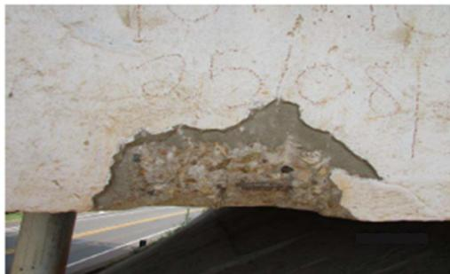
a) Longitudinal beam 3, on overhang 3, with crumbling concrete and exposed reinforcement
